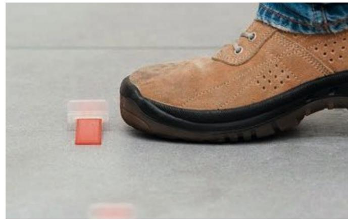
Once the adhesive cement has set, to remove the clip you simply need to tap it with the rubber mallet or the tip of your toe in the direction of the joint.
